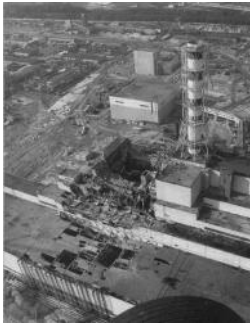
Fig.3. Nuclear power plant after the explosion.
