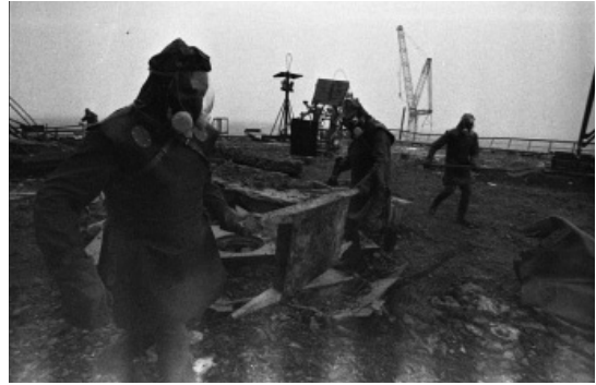
Fig.6 Firemen on the roof of the power plant.
