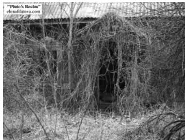
Fig.10 Abandoned house overgrown by vine
